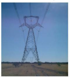
MAX HEIGHT = 40M WIDTH AT TOP = 17.2M WIDTH AT BOTTOM = 9M
